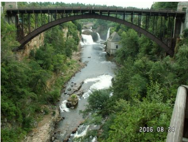
Ausable Chasm: The building below the arch of the U.S. Hwy. 9 Bridge houses turbines for a hydro-electric generating station. – Photo, Bob Lundy
