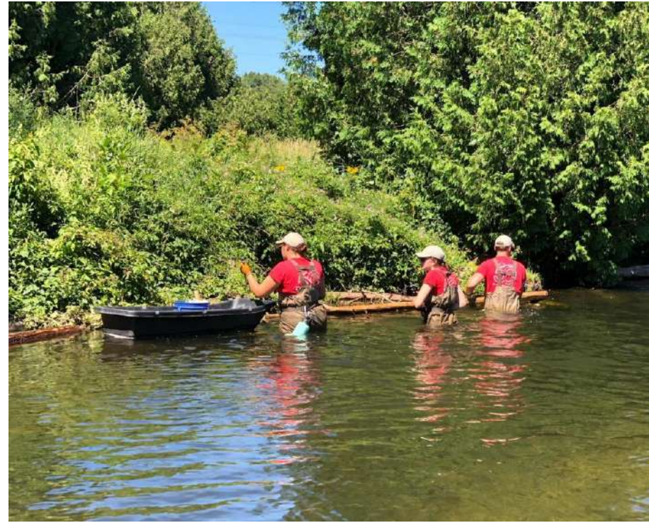
August 11 - Securing cedar logs in place to create additional habitat/refuge for brook trout
